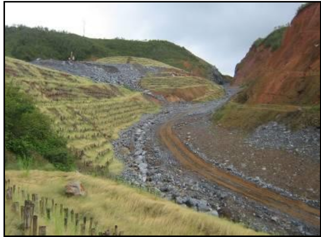
Ambatovy Pipeline project
